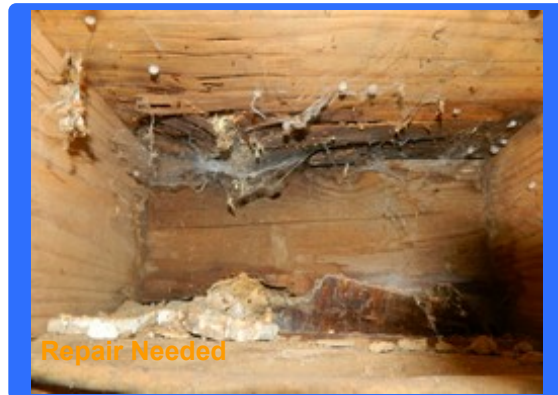
Termite damaged floor joists, band boards and subflooring. Recommend evaluation and repair by qualified contractor.
