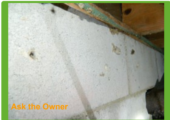
Evidence of past termite treatment observed. Recommend asking owner for more information and any transferable warranties.
