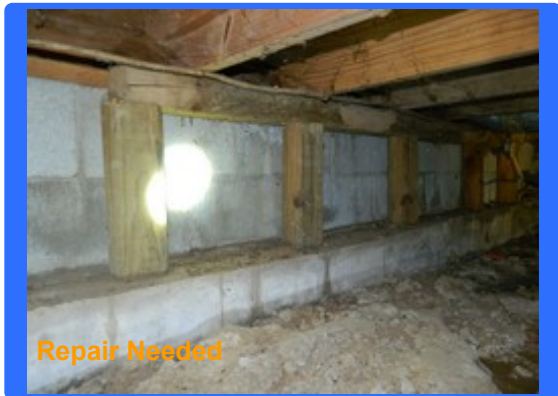
Substandard cribbing under floor joists. Band board and floor joists are deteriorated. Recommend evaluation and repair by qualified contractor.
