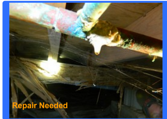
Copper piping in several areas was leaking. Suggest having a qualified plumber fully evaluate and make repairs.
